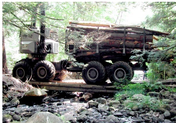
Figure 8-8 Temporary stream crossing
