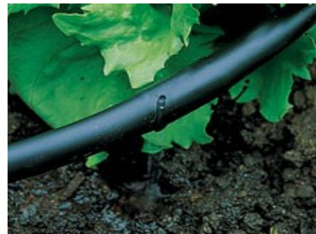
Figure 2-8 A drip system watering individual plant.
